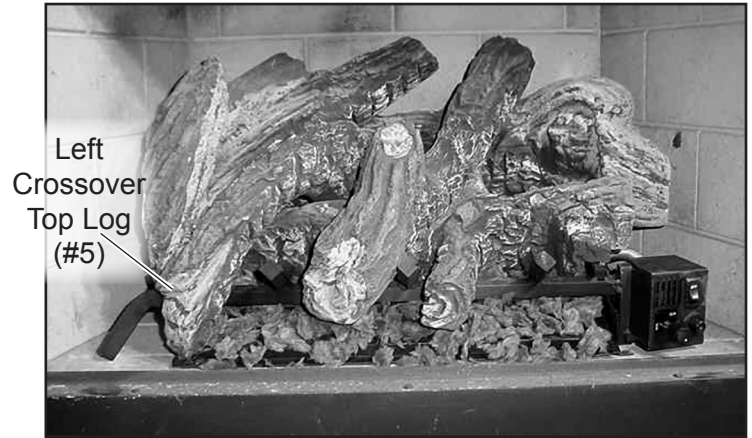
Figure 17 - Placing Left Top Log (#5)
