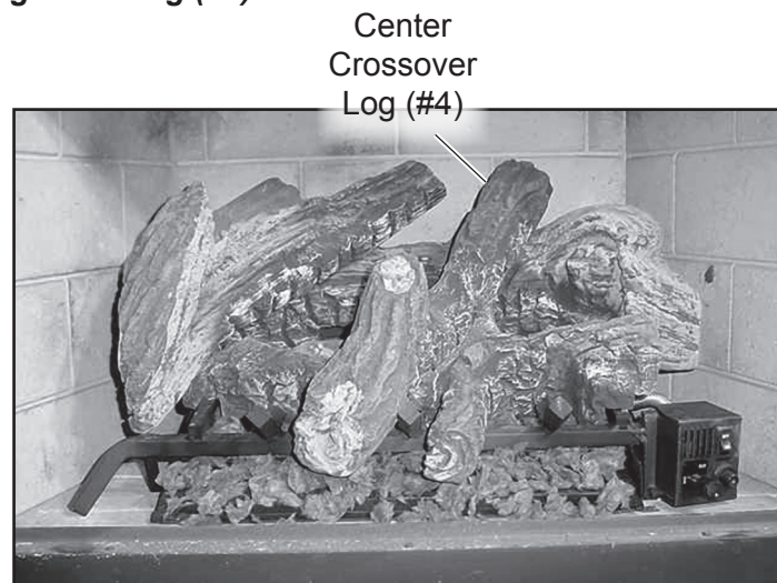
Figure 16 - Placing Center Log (#4)
