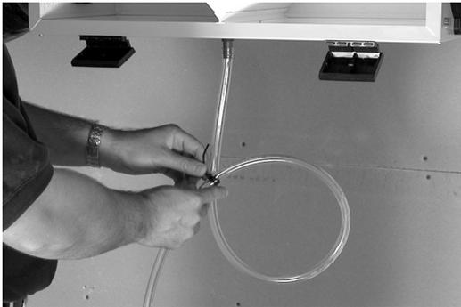
Make a loop in condensate line, not be subject to freezing temperatures.
