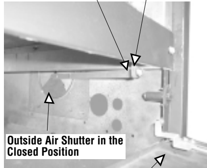
Control Compartment Access Panel Outside Air Control Lever and Securing Screw Location (EBVST, EBVPF and EBVCR Units Shown)
