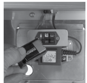
4. Insert and/or replace a new 9V battery
