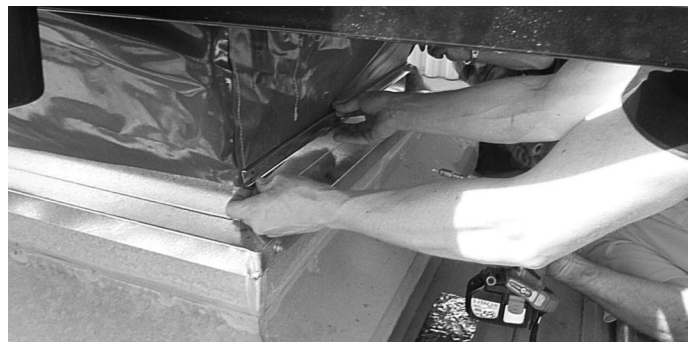
Fit the flexible duct transition to the duct dropper.
