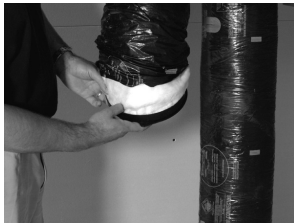
Insert insulation inside the double collar.
